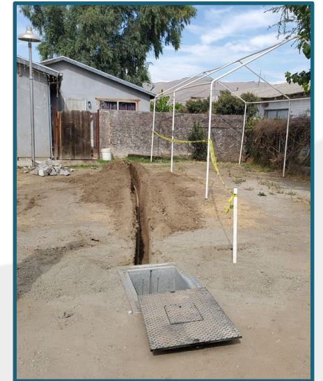
Photos: Seville Drinking Water Project
