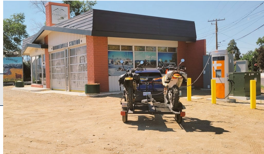
EV Charger and Welcome Center
