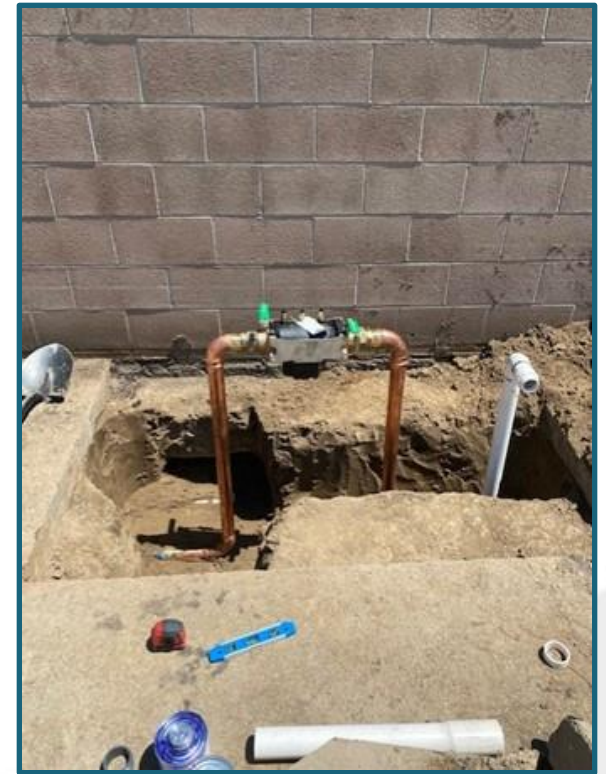
Photo: Del Rancho Y Emergency Funding for Interconnection
